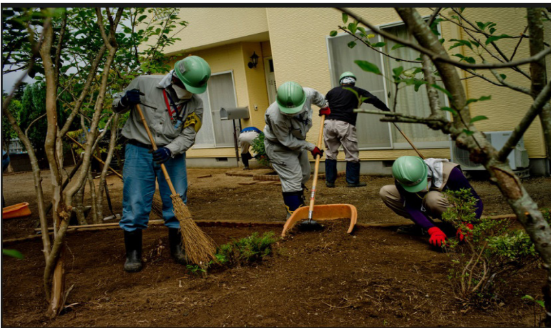
Workers removed the top soil of a garden from a house in Naraha. The national government hopes to eventually deploy an army of workers to scrape up tons of contaminated soil. But scouring the soil has had only limited success in bringing
