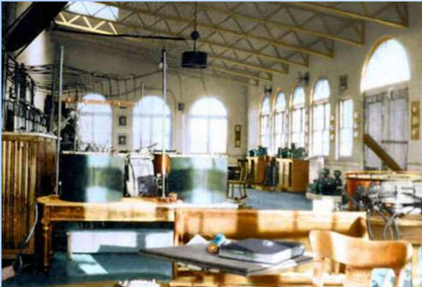
The interior appearance of the building-laboratory in Wardenclyffe in 1903. Left: the room for the experiments. Right: the workshop with the lathes and tools
