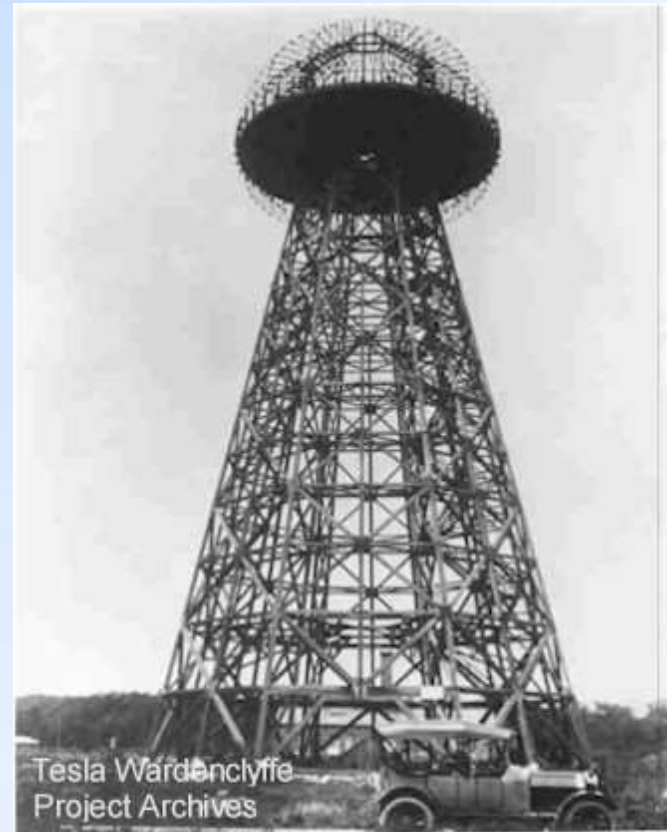
Wardenclyffe tower (Long island) in 1903 with the steel ribs without the copper sheath
