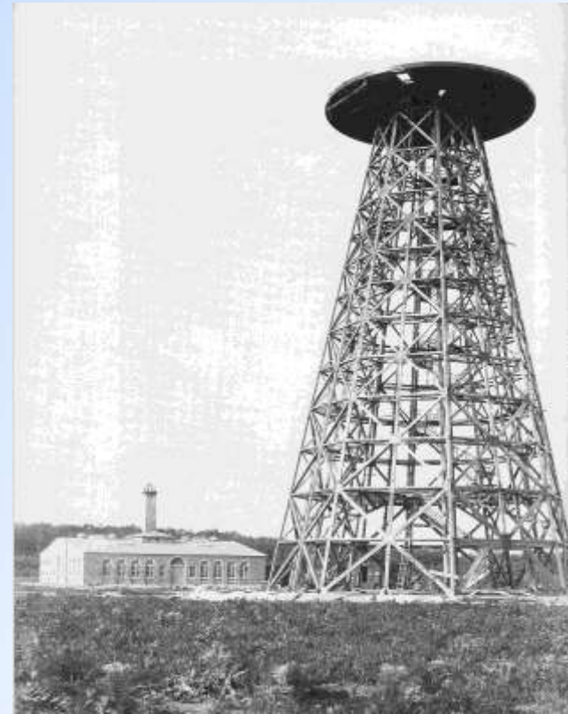
Wardenclyffe tower (Long Island) in 1902 with finished platform of the cupola
