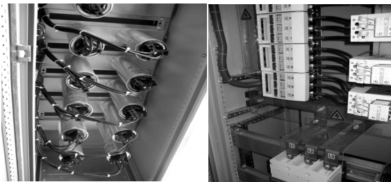
Fig. 5. Mechanical switched compensation system
