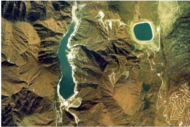
675 MW Numappara Pumped Storage Power Plant - Japonya
