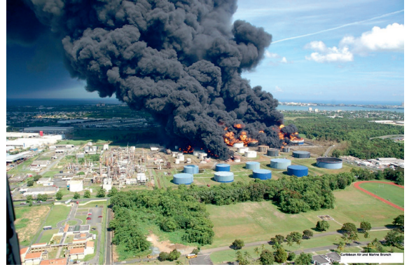
Görsel - Caribbean Petroleum Corporation (CAPECO) Refinery Tank Explosion and Fire (2009)
