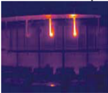
Blocked pipework
