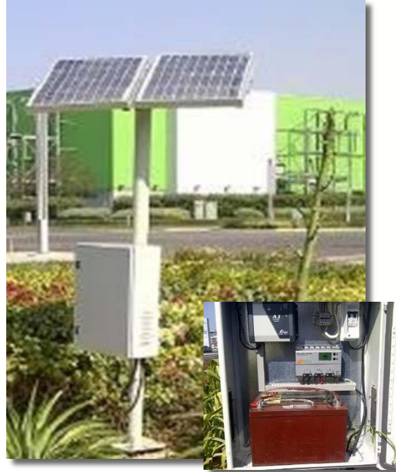
AGM 31 Solar street light in Dubai
