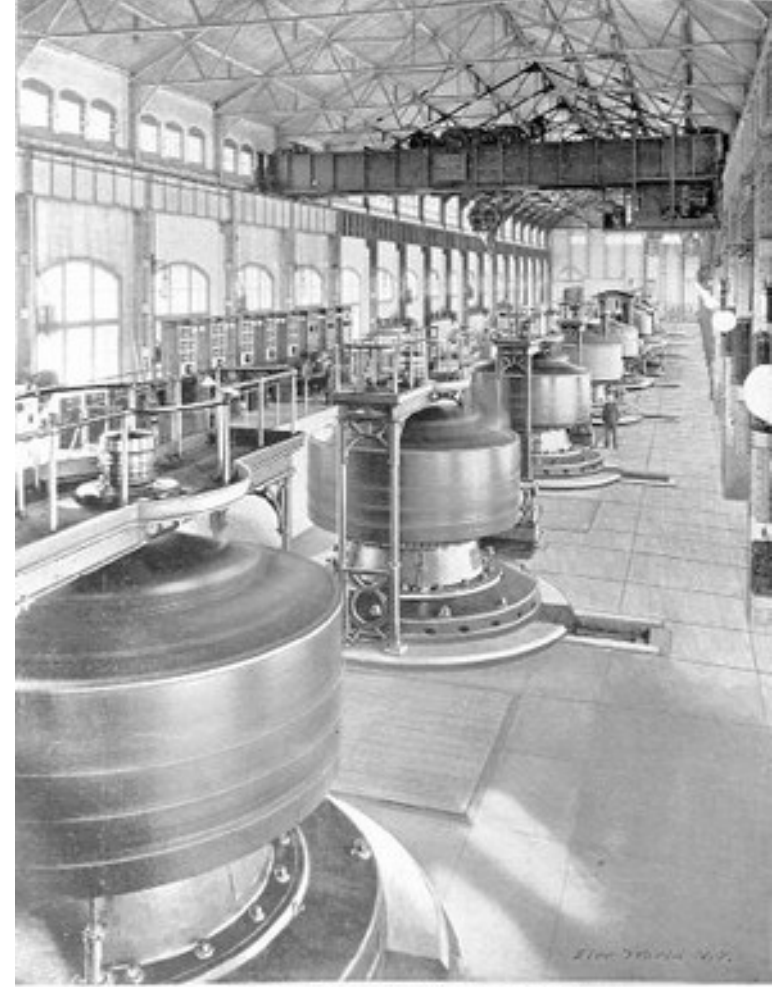
FIG. 41-10 VIEW OF THE TURBINE ROOM, LOOKING SOUTH FROM THE VISITORS' GALLERY.
