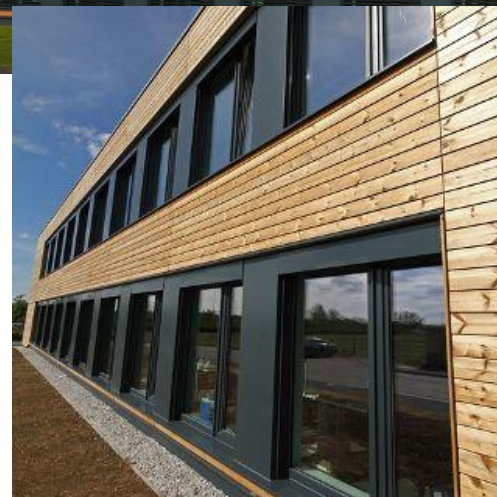
REHAU GENEIO® window (Uf= 0.91, Ug= 0.5, window size 123 x 148 cm
