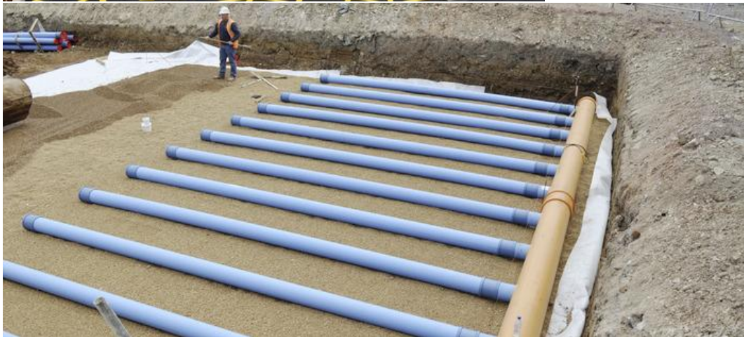
REHAU AWADUKT Thermo ground – air heat exchanger
