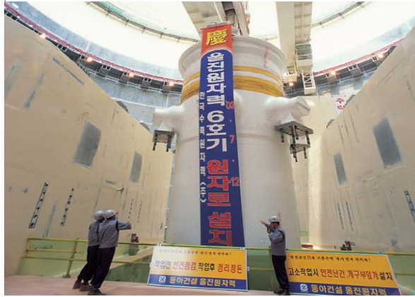
Installation of Reactor Vessel KORE-Reaktör Montajı
