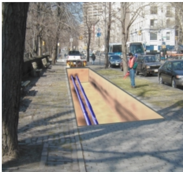
Fig. 1 Underground Transmission lines detected by GPiR
