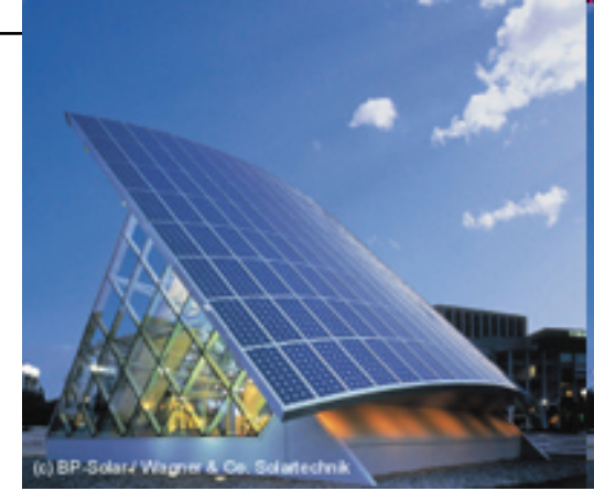
BP solar, energy park, İngiltere
