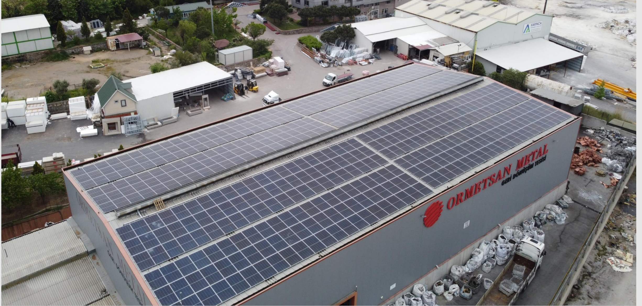
Ormetsan Metal Gebze/Kocaeli 287,76kWp/240kWe
