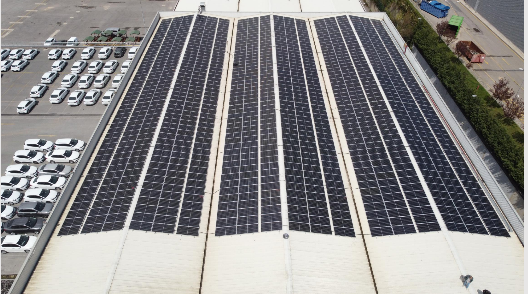
Coil Partners Çayırova/KOCAELİ 409,5kWp/400kWe
