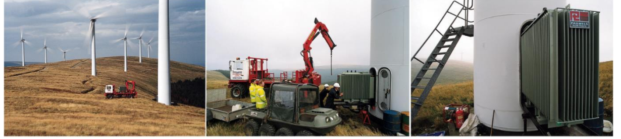
NEG-MICON 630kVA 30kV fused
