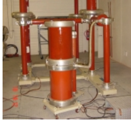
Figure 1: Photograph of the cascaded AC transformers
