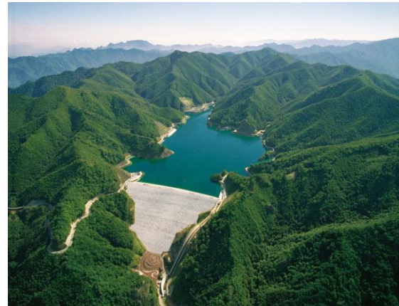
2700 MW Kannagawa Pumped Storage – Japonya -2005
